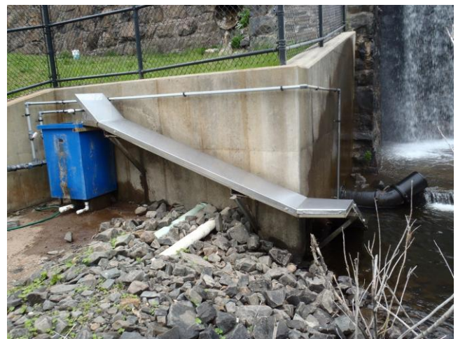
The Mill River Eel Pass was recently rehabilitated by its owner, the Southcentral Regional Water Authority. This is a blind eel pass in which eels are collected in the blue tank and carried over the dam.
