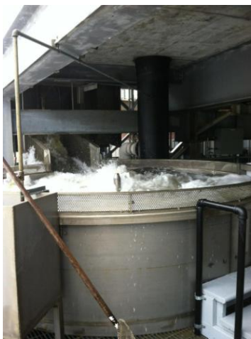
The holding tank at Holyoke Dam receiving the contents of a hopper lift. Most lifts discharge at the next level up where the fish swim out to continue their migration. When we want to truck shad, we discharge into this lower tank where fish can be diverted into transport trucks.
